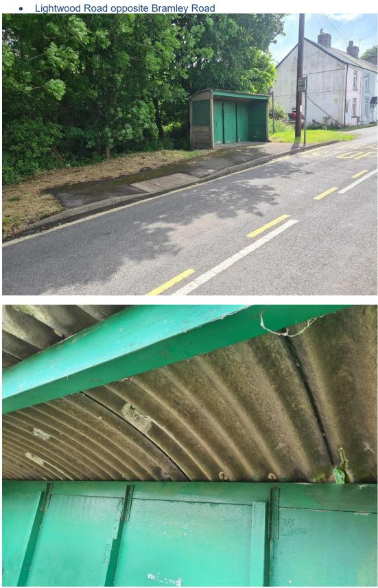
The roof of this older shelter is in a very poor state with holes in what appears to be an concrete/asbestos ridged panel roof, the shelter and boarding point also fail to meet latest accessibility standards.
